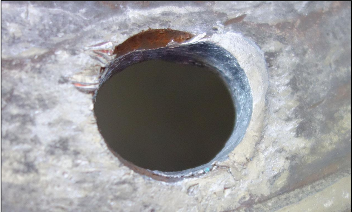
Photograph 5: Outer wheel stud hole damage
