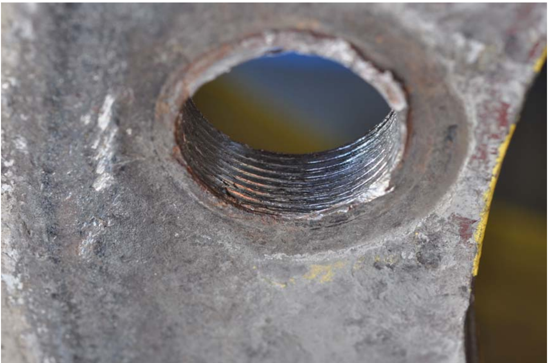
Photograph 2: Damaged Inner Rim Stud Hole
