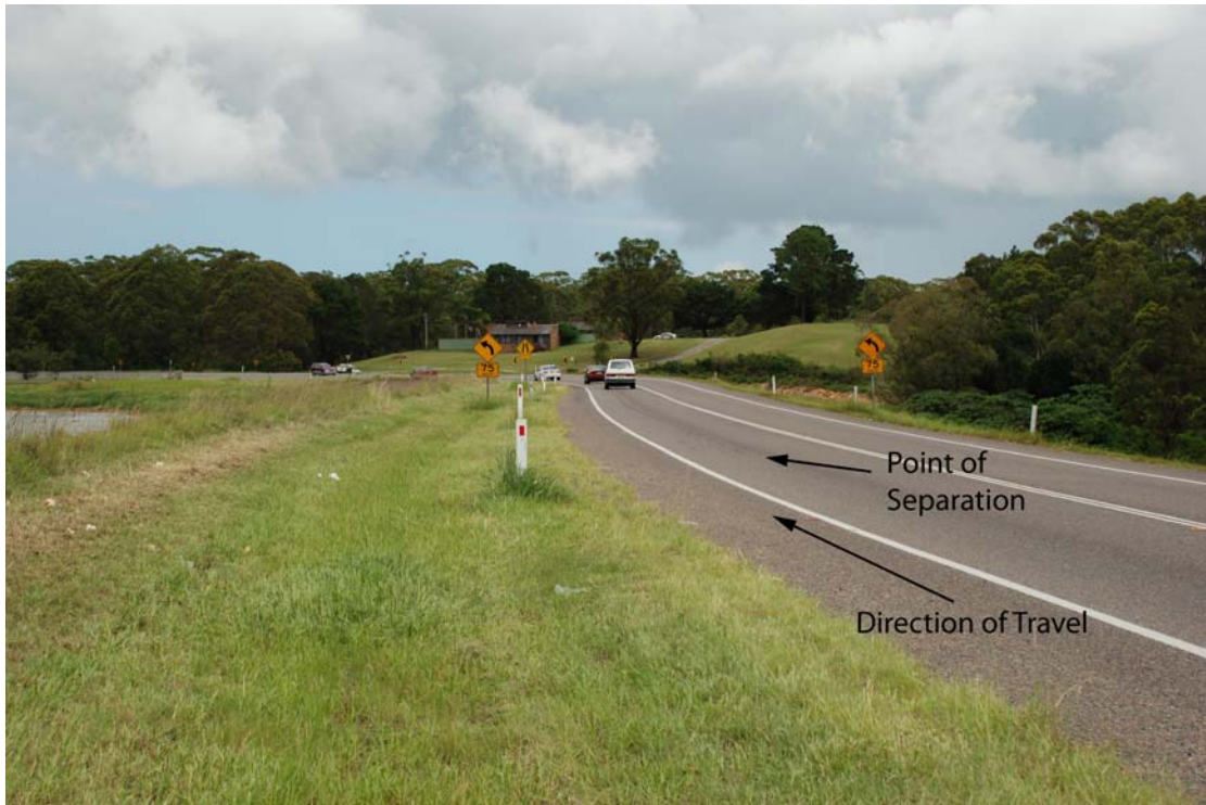
Photograph 10: Road Conditions at Point of Separation
