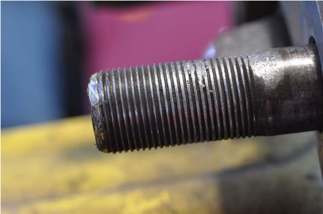
Photograph 3: Example of Stud Damage
