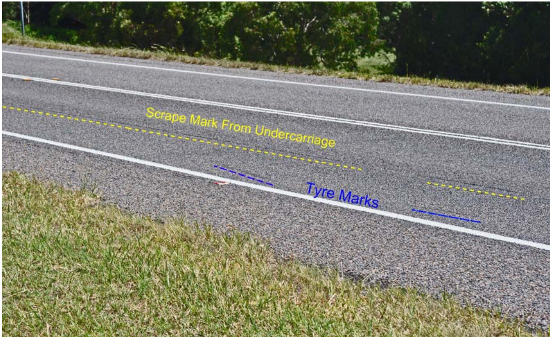
Photograph 8: Scrape and Tyre Marks on Road
