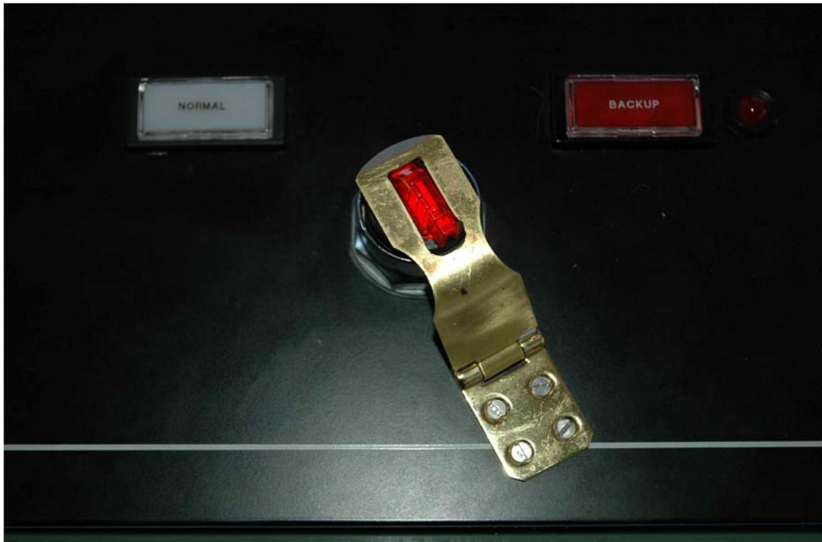
**Figure 8: Retro-fitted 'Lockout' on Normal-Backup Mode Switch**
