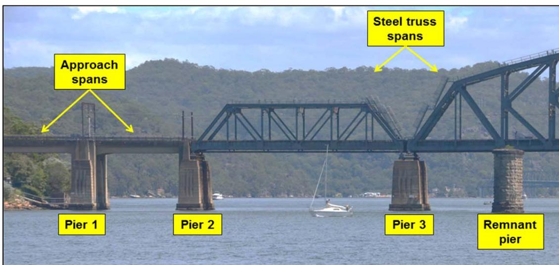
Photograph 2: Southern end of bridge showing piers and spans
