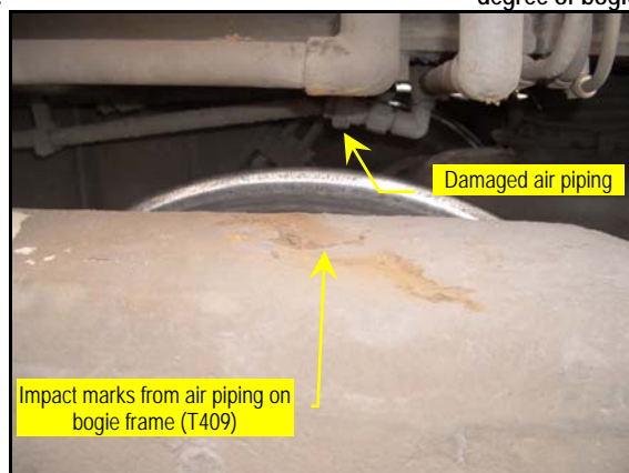
Photo 5: Impact marks on leading bogie and damage to piping of air brake system of T409
