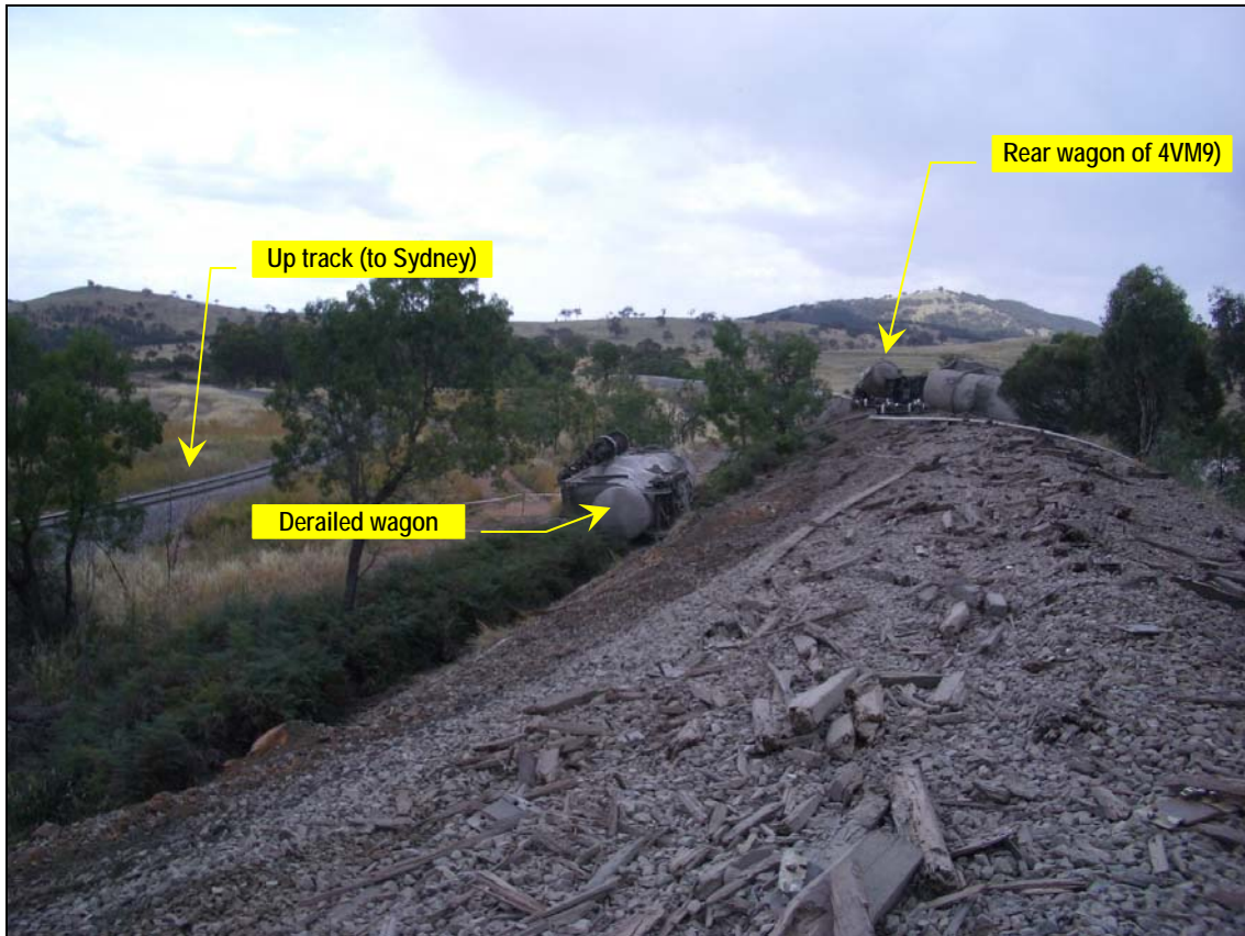
Photo 6: Incident site looking towards Sydney showing extent of track damage.
