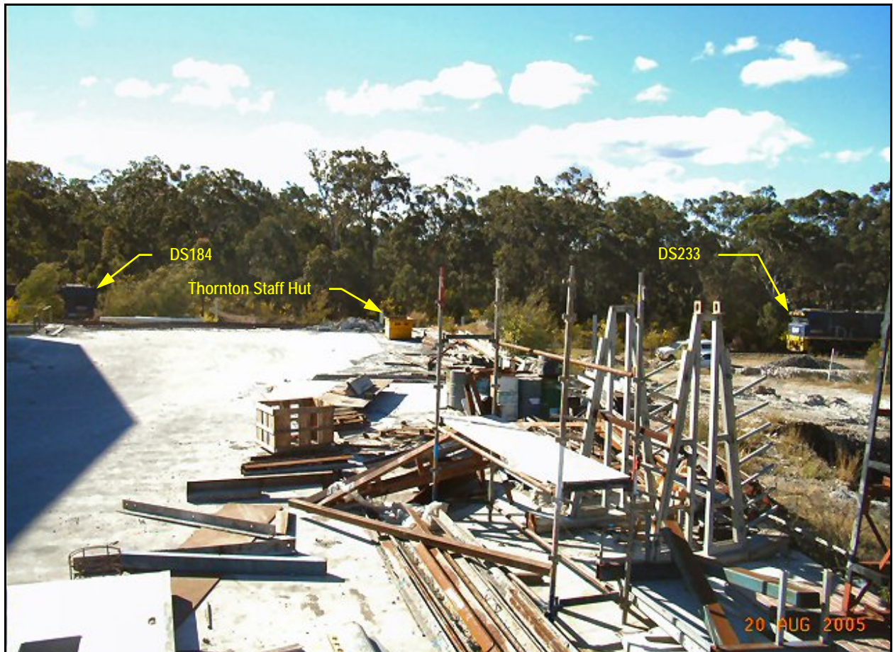
Photograph 1: Relative Positions of DS233 to DS184 after the Incident (Photo supplied by ARTC)
