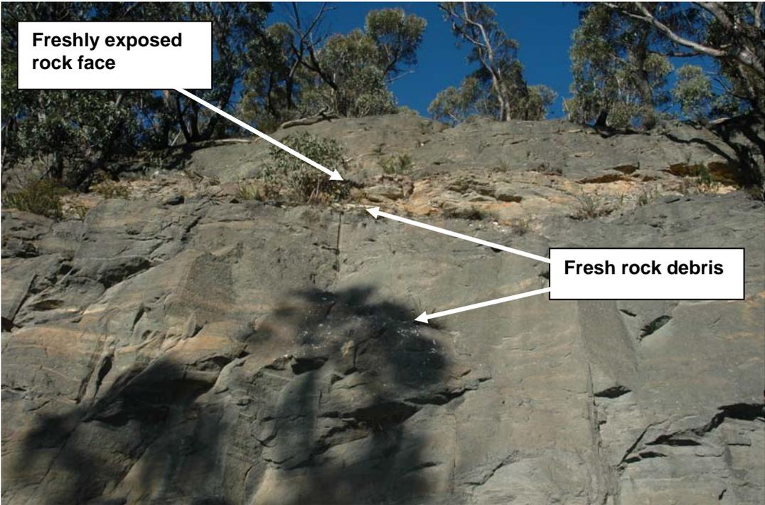
Figure 3 –View of Rock Face and Associated Debris
