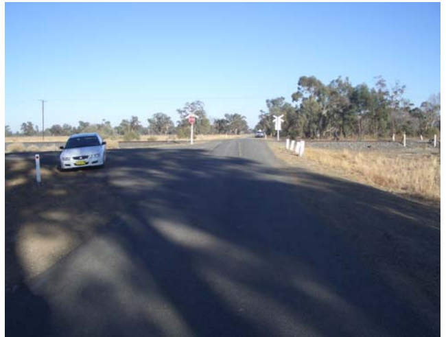
Photo 9: View of, and 50m from, the level crossing
