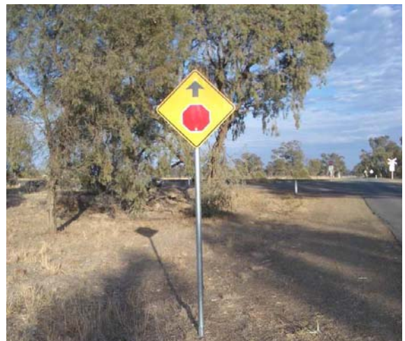
Photo 15: Warning sign post-accident
