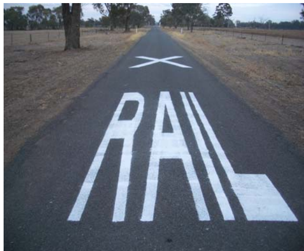
Photo 14: Road marking post-accident
