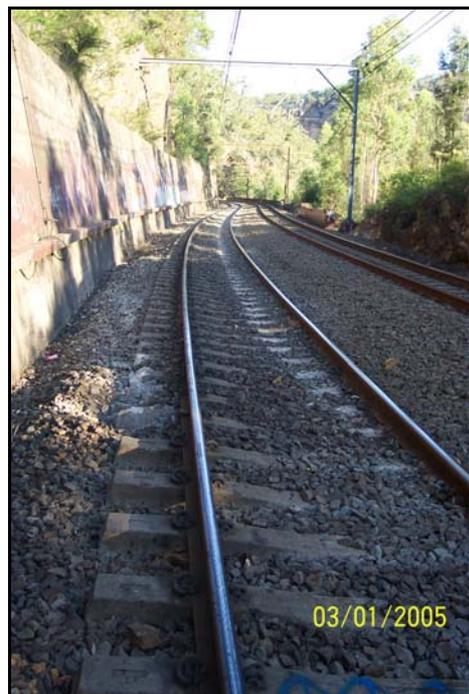
Photo 7 Commencement of Sleeper Damage at Lapstone
