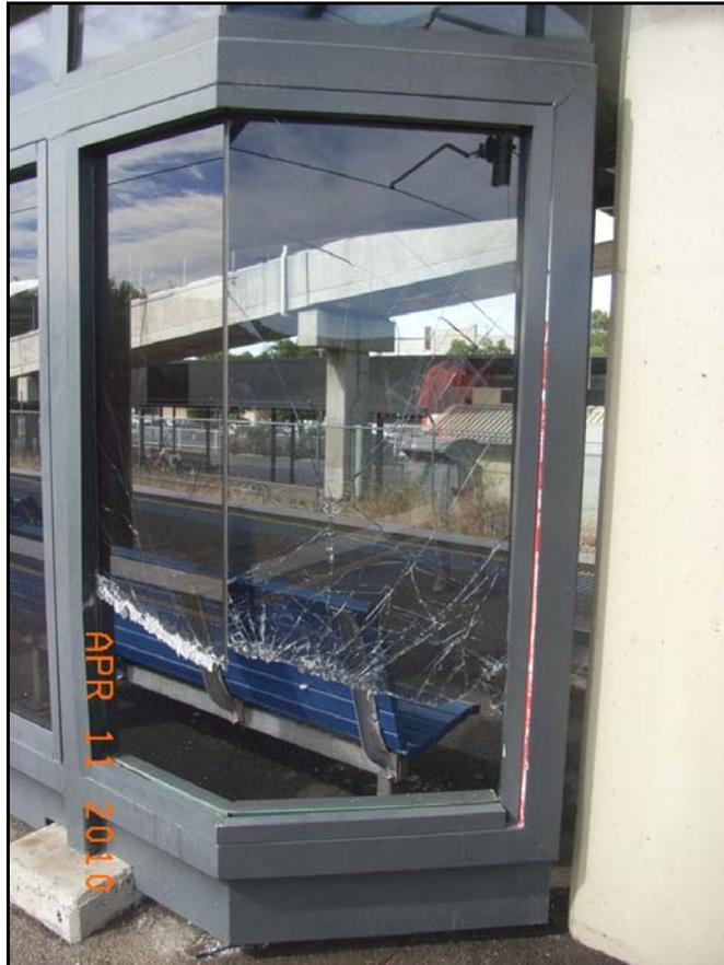
**Photograph 4:** Broken glass on seating bay windbreak
