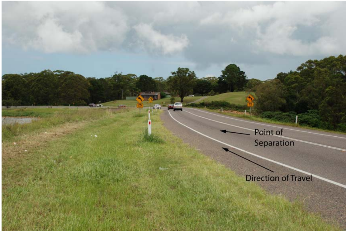
Photograph 10: Road Conditions at Point of Separation
