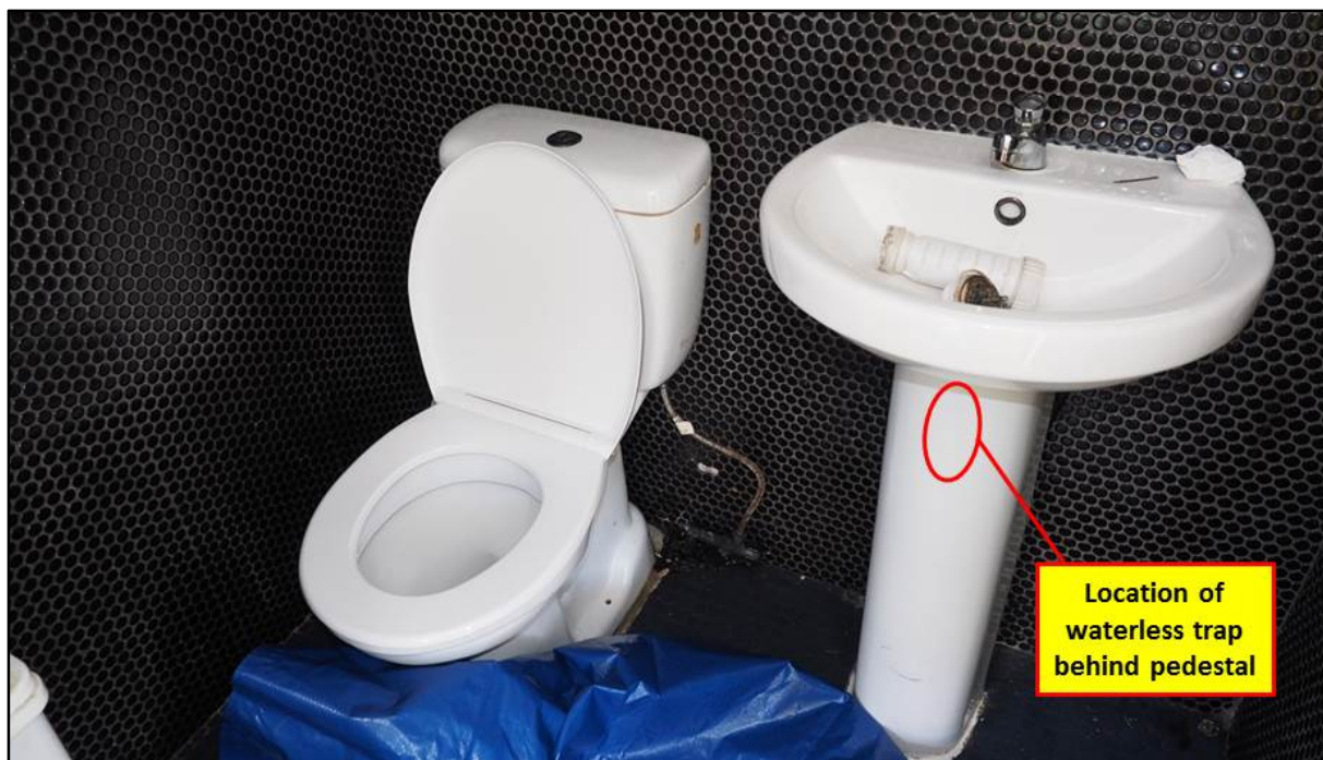
Figure 16: Location of waterless trap behind basin pedestal
