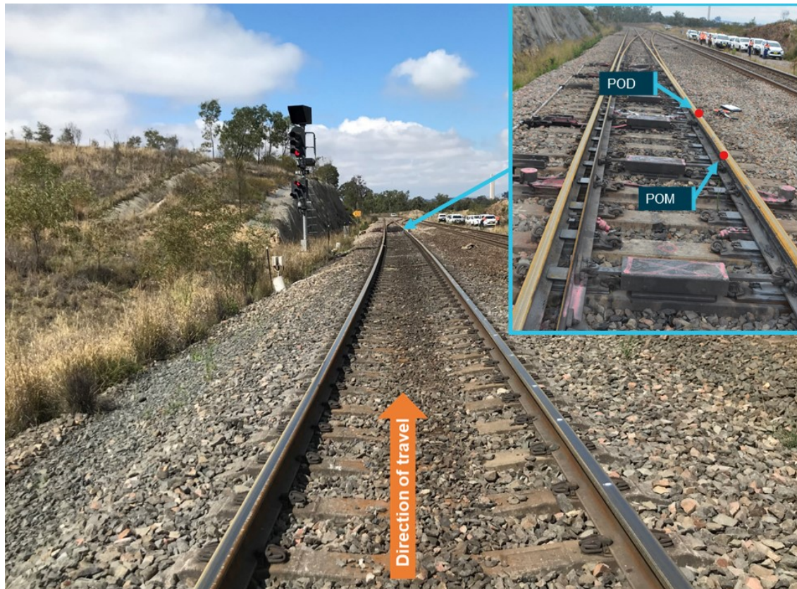
Figure 7: Point of Mount (POM) and Point of Dismount (POD) – Antiene Up direction
