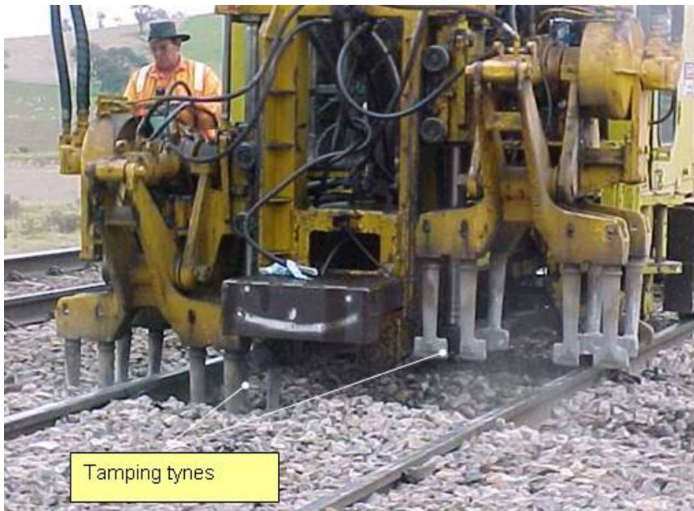
Figure 5 – Spot Tamping operation- front view
