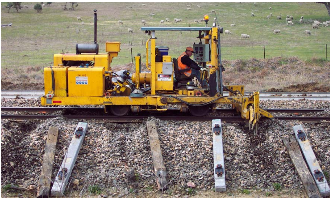
Figure 4 – Linear Scarifier (scarifying to install low profile concrete sleepers)
