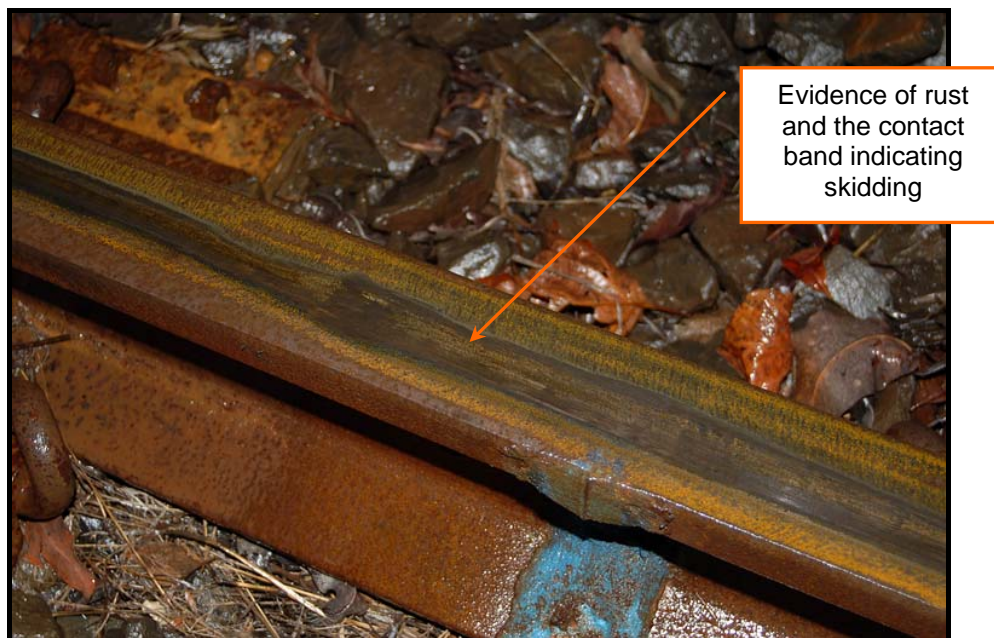
Photo 7: Evidence of rust emulsion and skid marks on the railhead.
