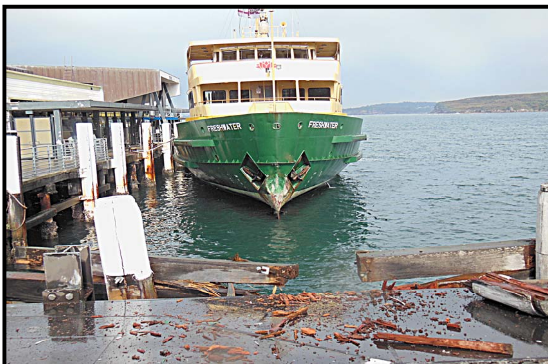
Photograph 3: Damage from the collision
