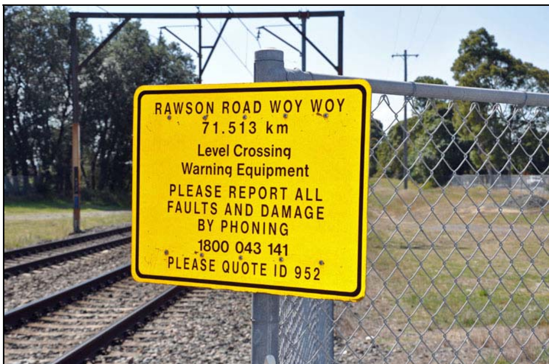
Photograph 13: Information signage for reporting defective level crossing equipment
