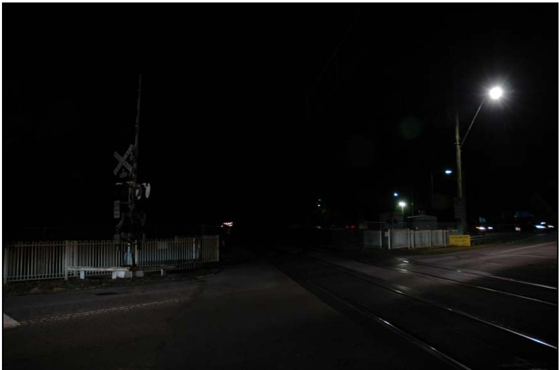
Photograph 2: Level crossing area where RMV driver entered rail corridor
