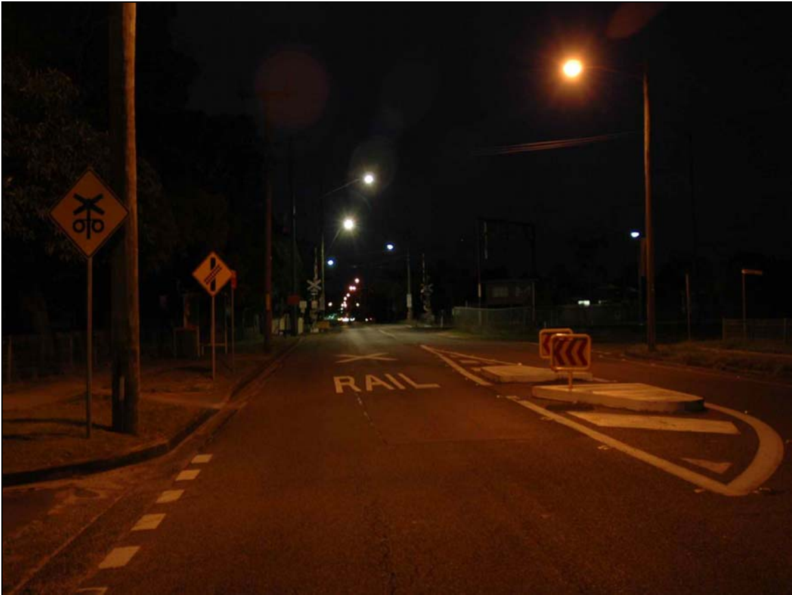
Photograph 12: Night time view of approach signage and pavement marking
