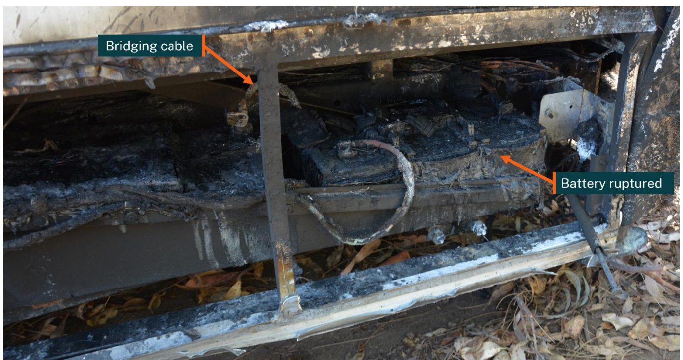
Figure 1: Umina Beach bus fire battery compartment
