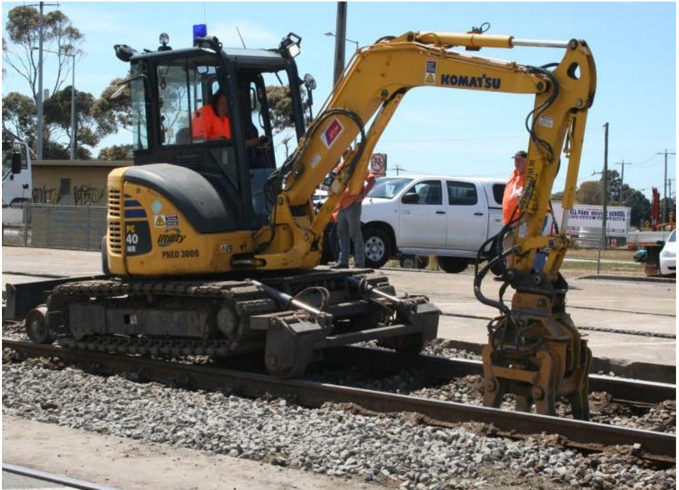
Figure 4: Example of rail mounted excavator with tamping attachment
