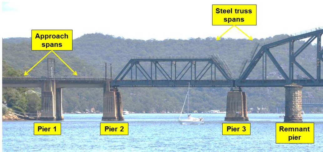
Figure 27: Southern end of bridge showing piers and spans.
