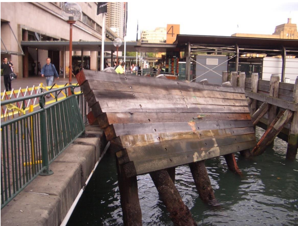
Figure 11: Damage from Freshwater class vessel Collaroy collision at Circular Quay.
