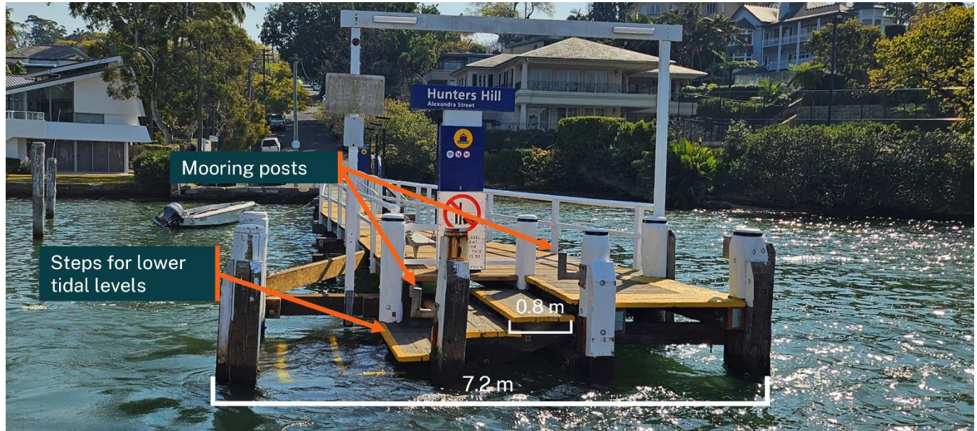
Figure 36: Hunters Hill Wharf – fixed structure
